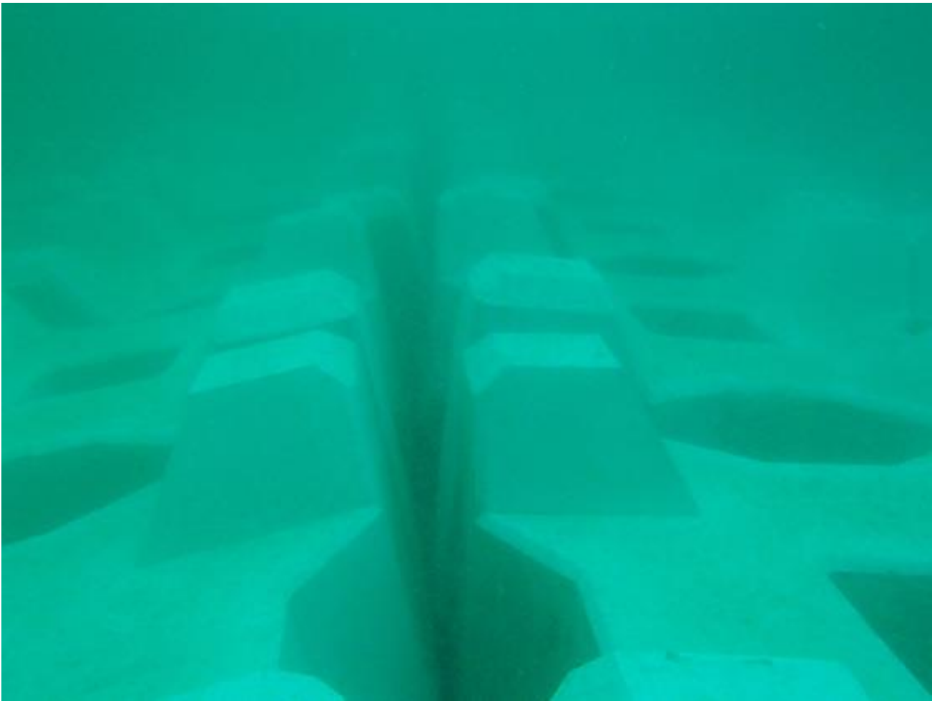
Installed foot protection block
