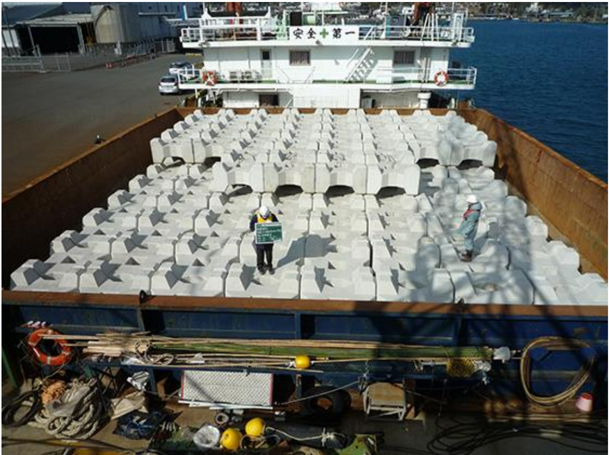
Foot protection blocks loaded on vessel
