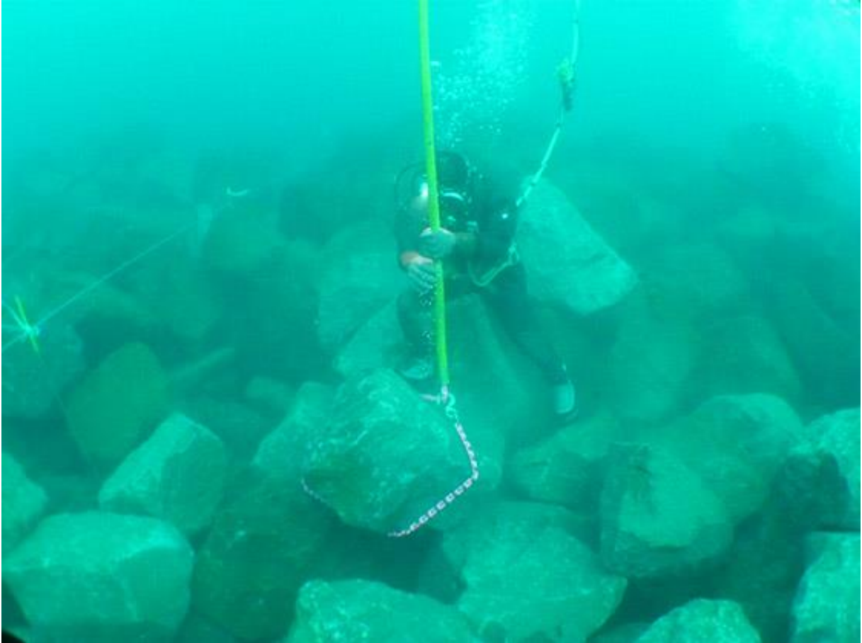
Heavy objects are moved using a diver boat's winch
