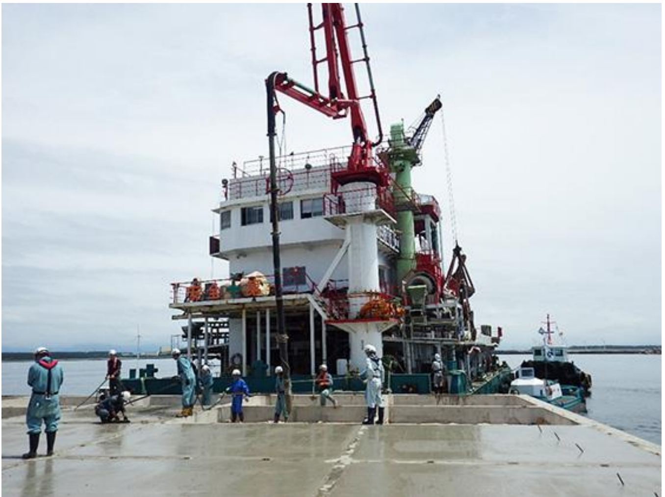
Laying lid concrete
