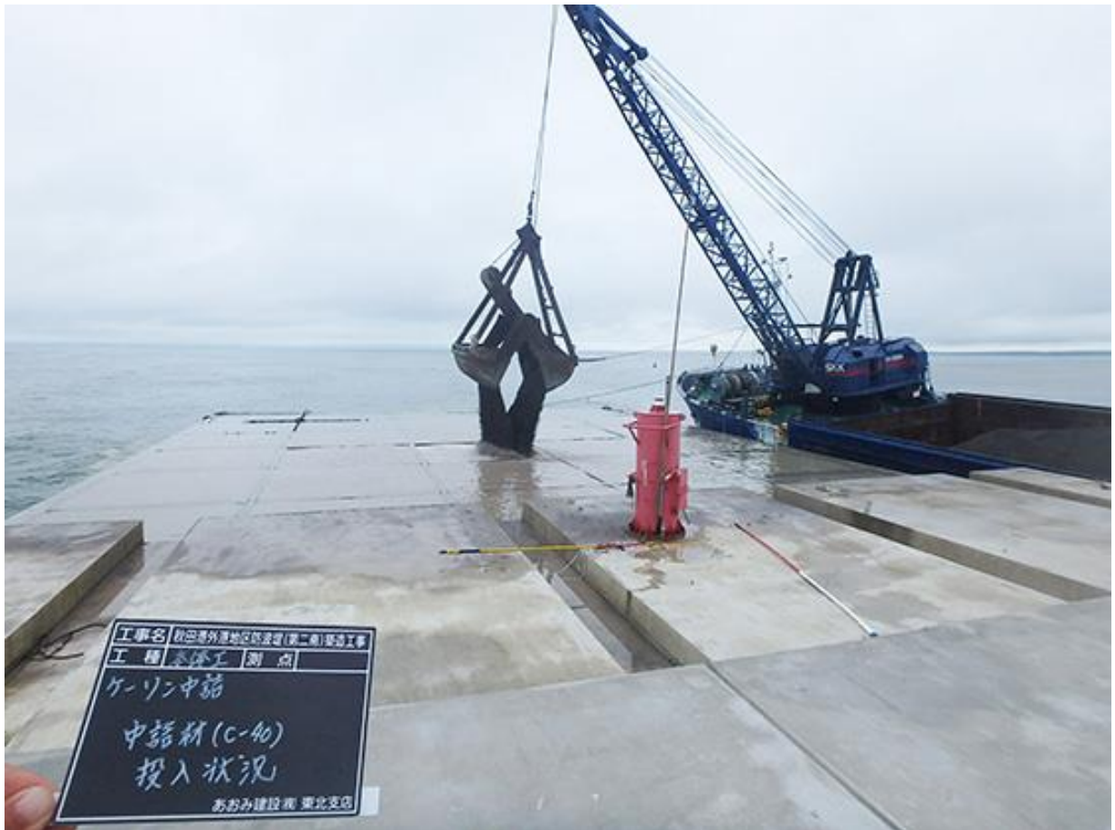
Filler material inserted
