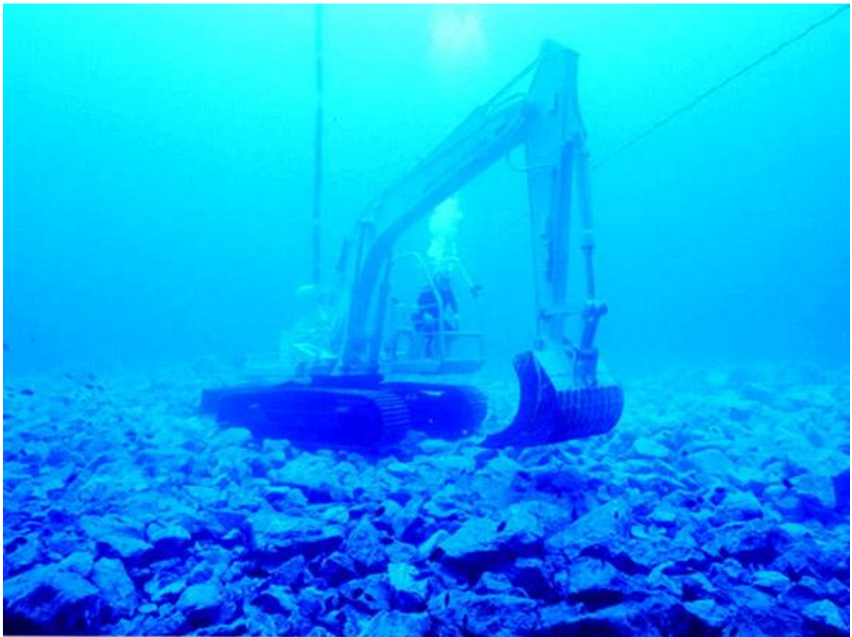
Flattening work using an underwater backhoe and big club
