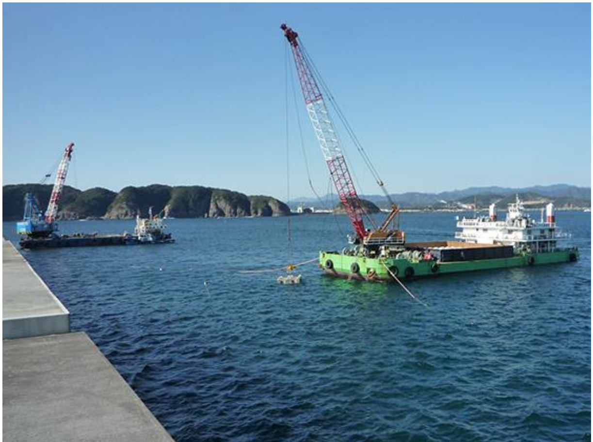
Foot protection block installation work
